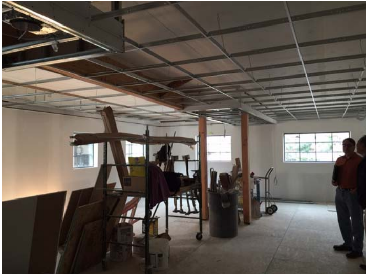
South and west walls— and new windows!
